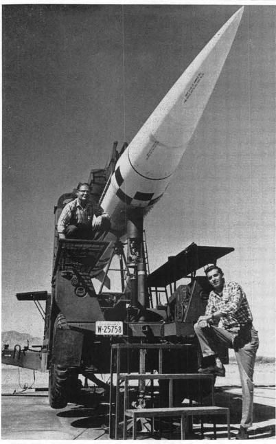
THE SERGEANT is a U.S. Army missile 31 inches in diameter and about 35 feet long. The missile's launcher is carried on a semitrailer. With the missile are Ed Stout (upper left) and Cal Cox.
